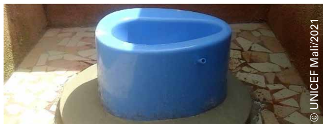
Disability-accessible toilet built locally using a SATO stool in the Sikasso region of Mali.
