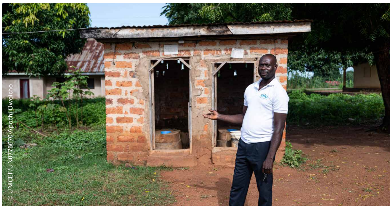
Kasua Tyolumun Moses, a toilet business entrepreneur who has participated in UNICEF-sponsored training sessions, sells SATO pans and other materials, and has installed over 600 toilets in Benue, Nigeria.
