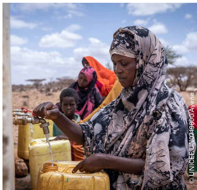
A woman draws water from a newly-installed water system in the drought-affected region of Ainabo in Somaliland. The system was constructed by UNICEF with funding from the United States of America.
