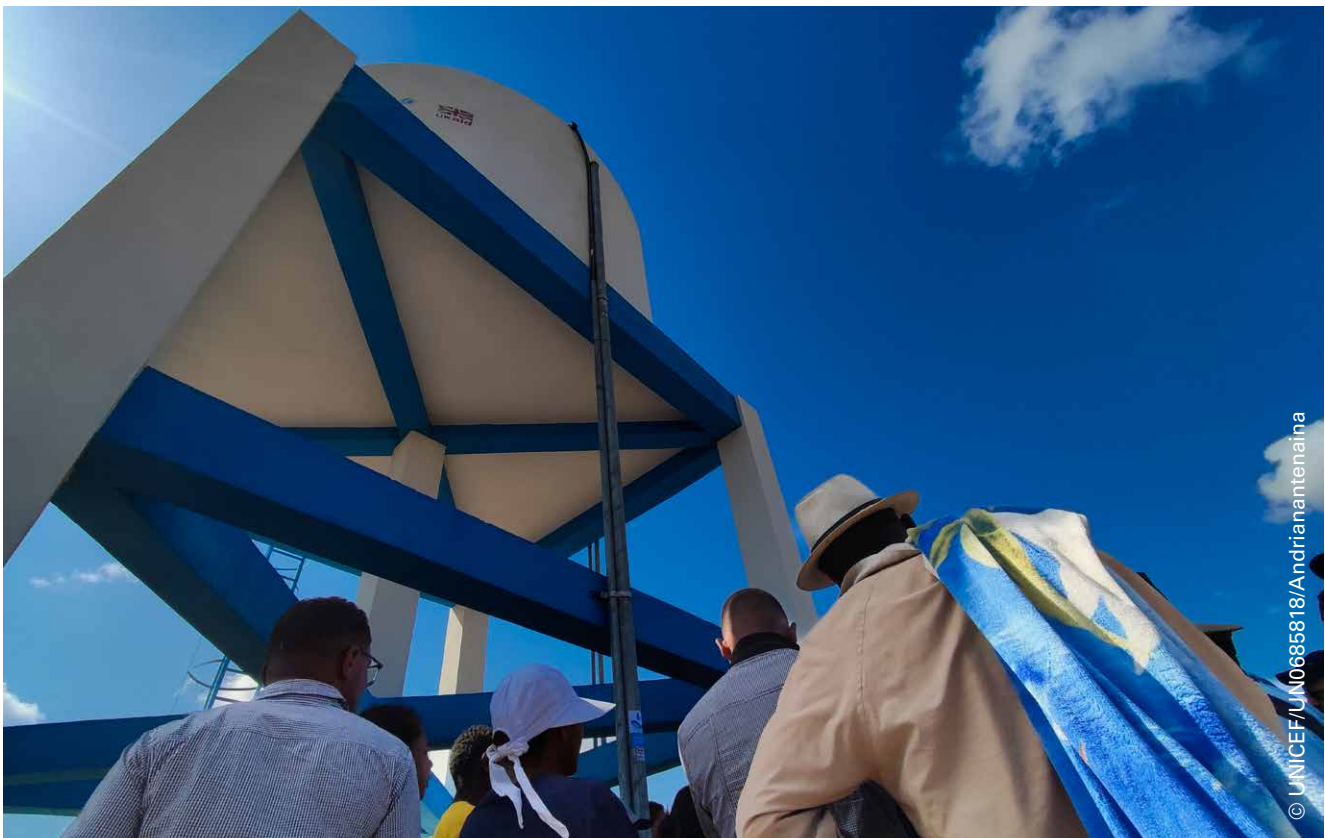
The water tank of a new solar-powered water system in the community of Androimpano, southern Madagascar, constructed by UNICEF with the support of the Government of the United Kingdom.
